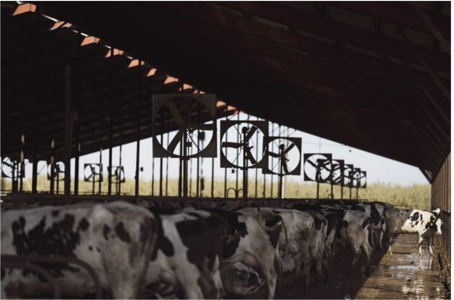
The cattle at Tom Barcellos' farm are kept cool with fans and misting machines. Photographer: Eric Thayer/Bloomberg
